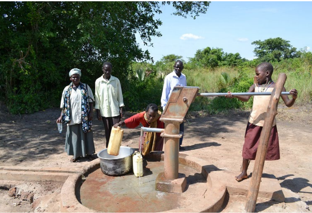
Boreholes constructed in Uganda to improve water infrastructure.
